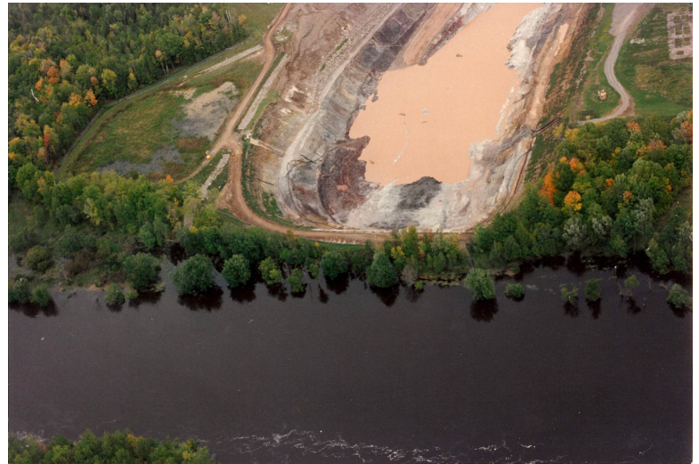
Flambeau Mine after river flooding showing the pit within 20 feet of the river Photo Credit: Bob Olsqard
